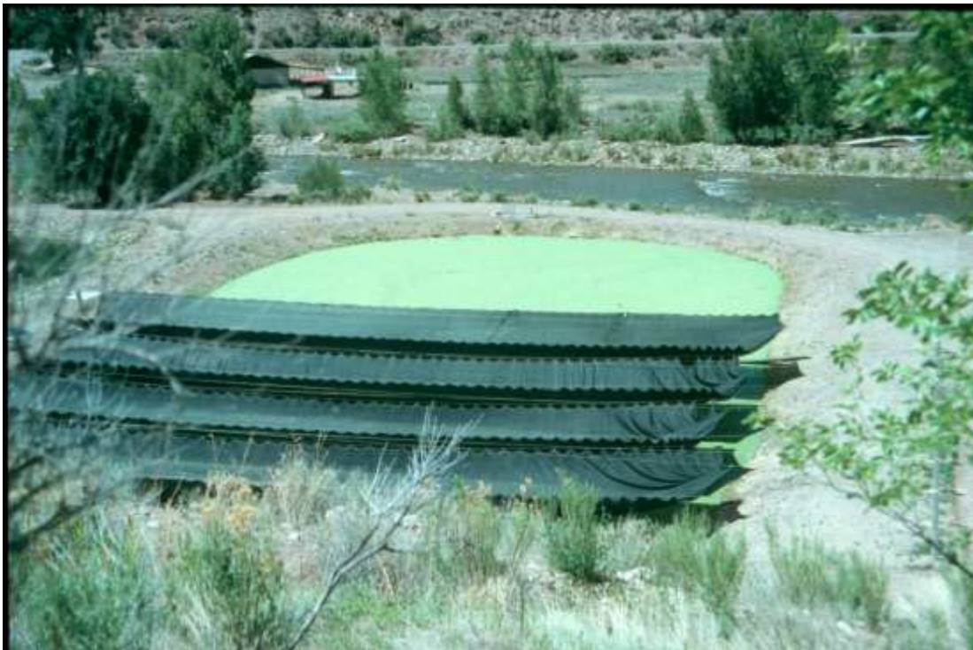
Figure 7-10. Photograph of shading for control of algal growth in Naturita, Colorado (R. Bowman, pers. comm., 2000).
