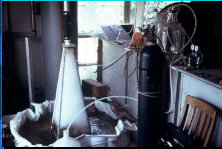
Figure 5-57. Photograph of the laboratory experiment used to develop the concept of the Speece Cone (Dominick and DeNatale, 2009).
